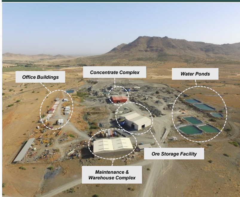
Kharrouba Complex Plant
